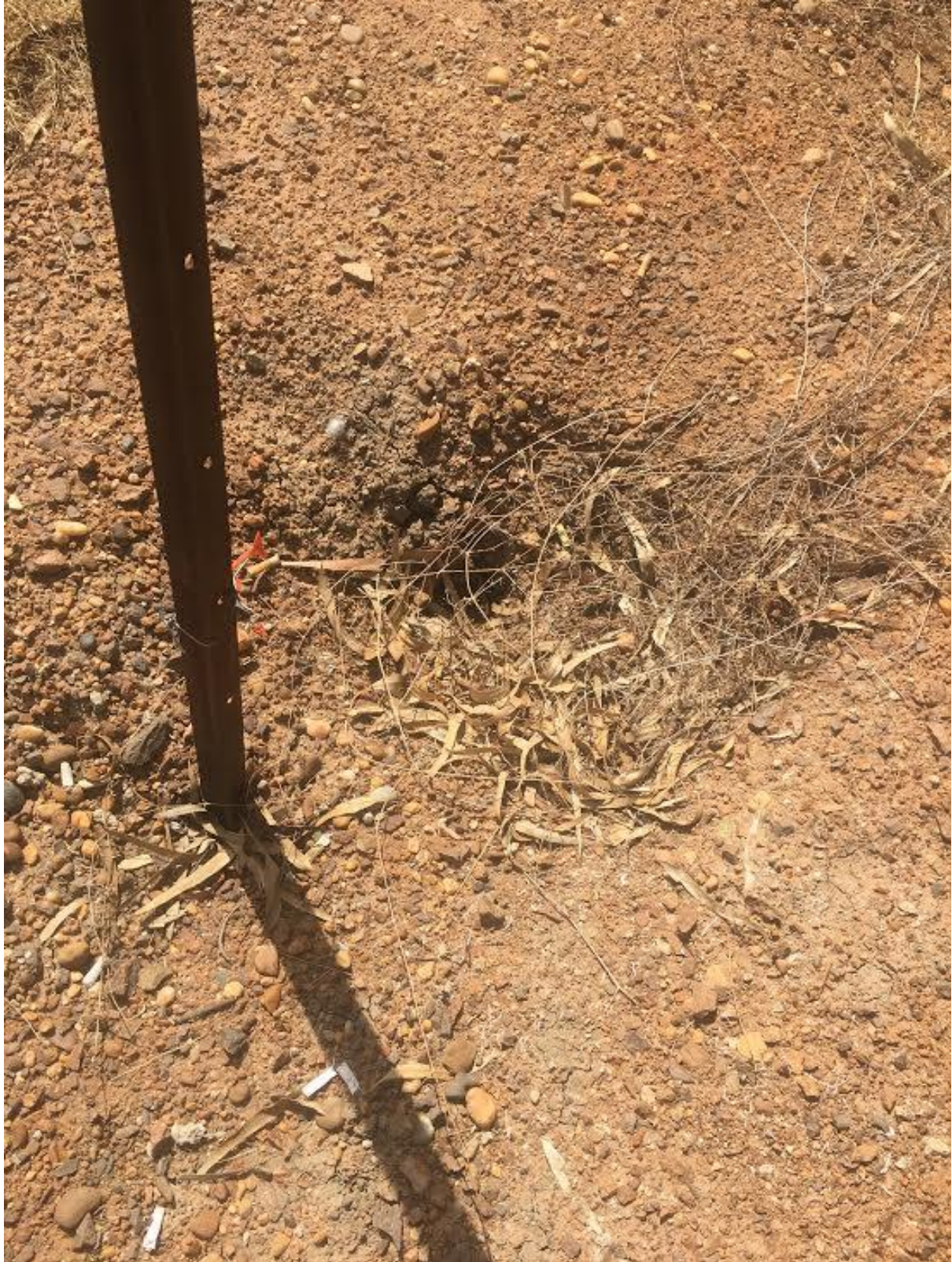
Photograph 9 Dentist Surgery/Courthouse piping
