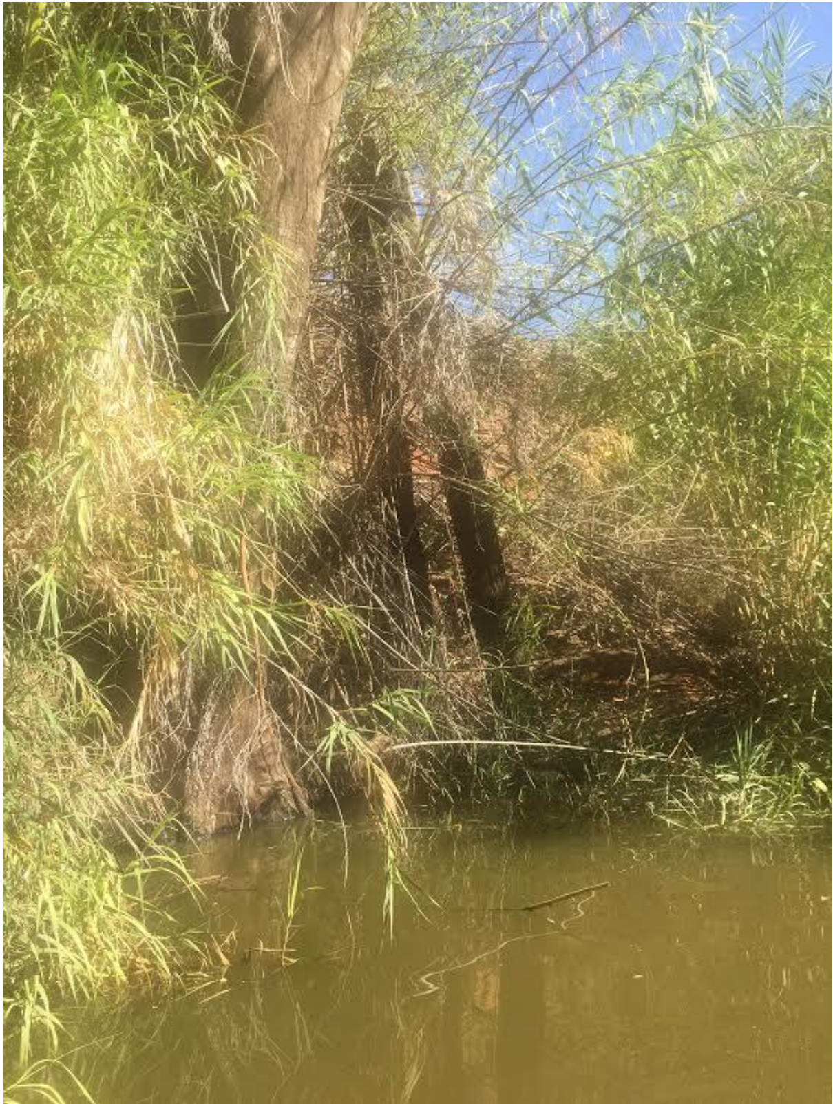
Photograph 4 Dentist Surgery/Courthouse Slippage - Old Wharf
