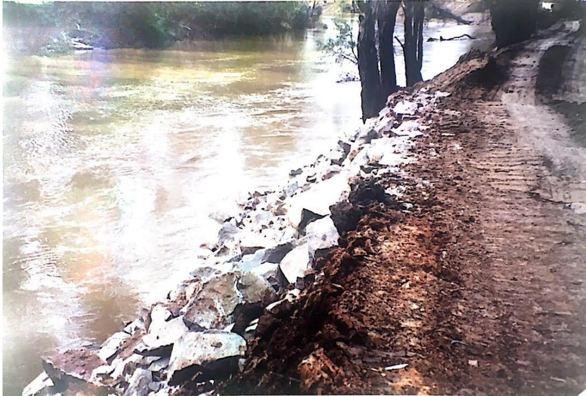
Photograph 23 Typical Levee Construction Riverside
