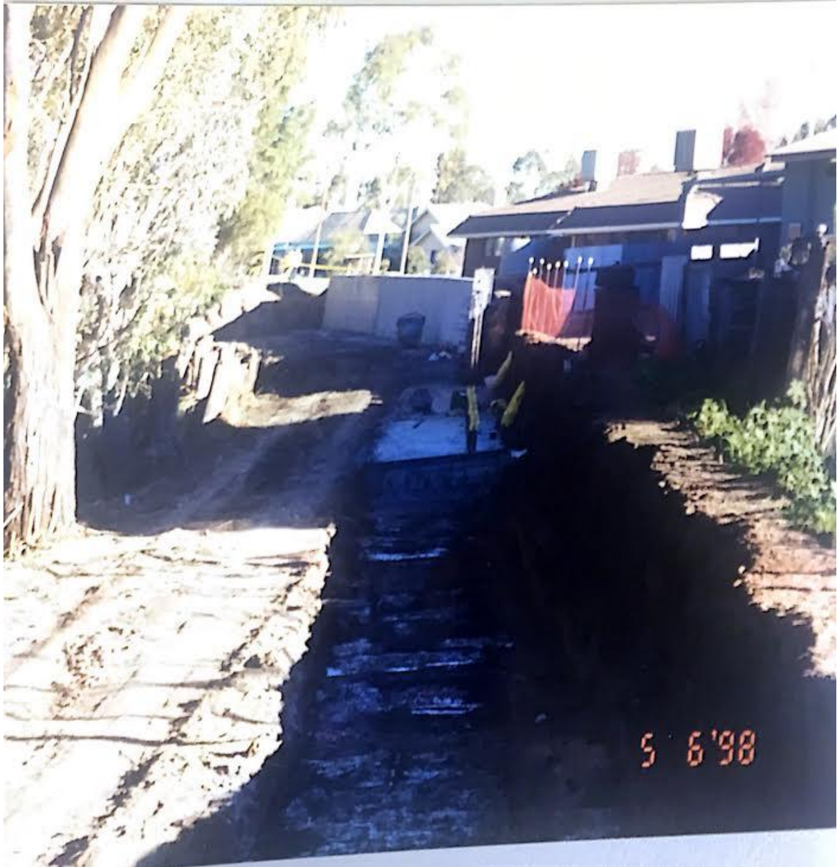
Photograph 19 Dentist Surgery/Courthouse Retaining Wall Construction
