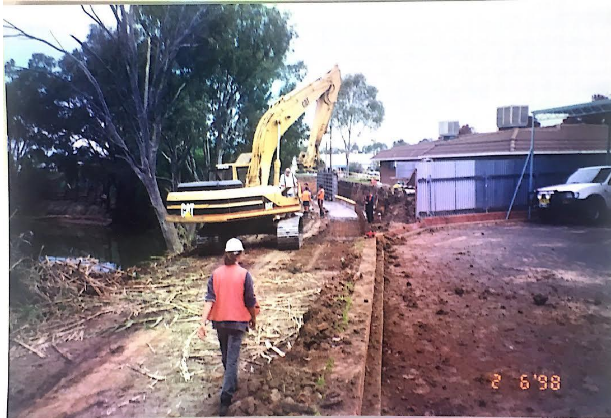
Photograph 18 Dentist Surgery/Courthouse Retaining Wall Construction
