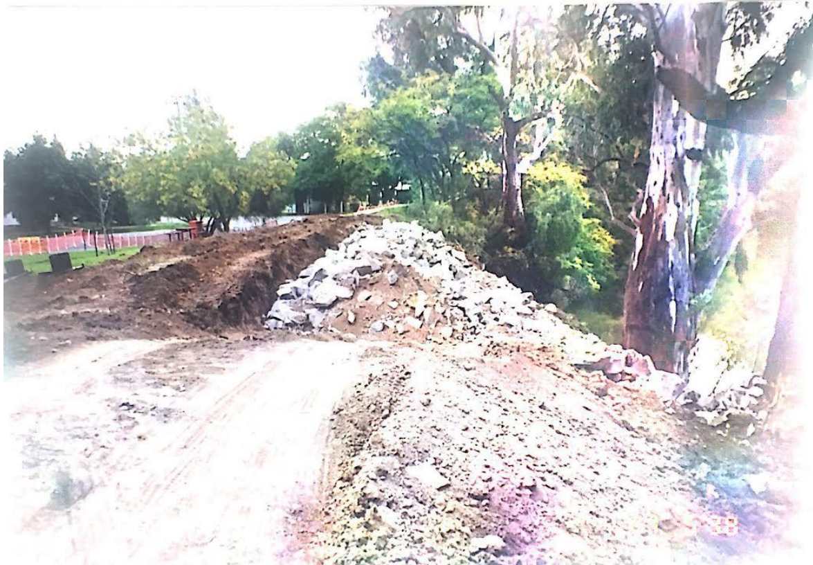
Photograph 24 Typical Rock Protection of Levee Riverside
