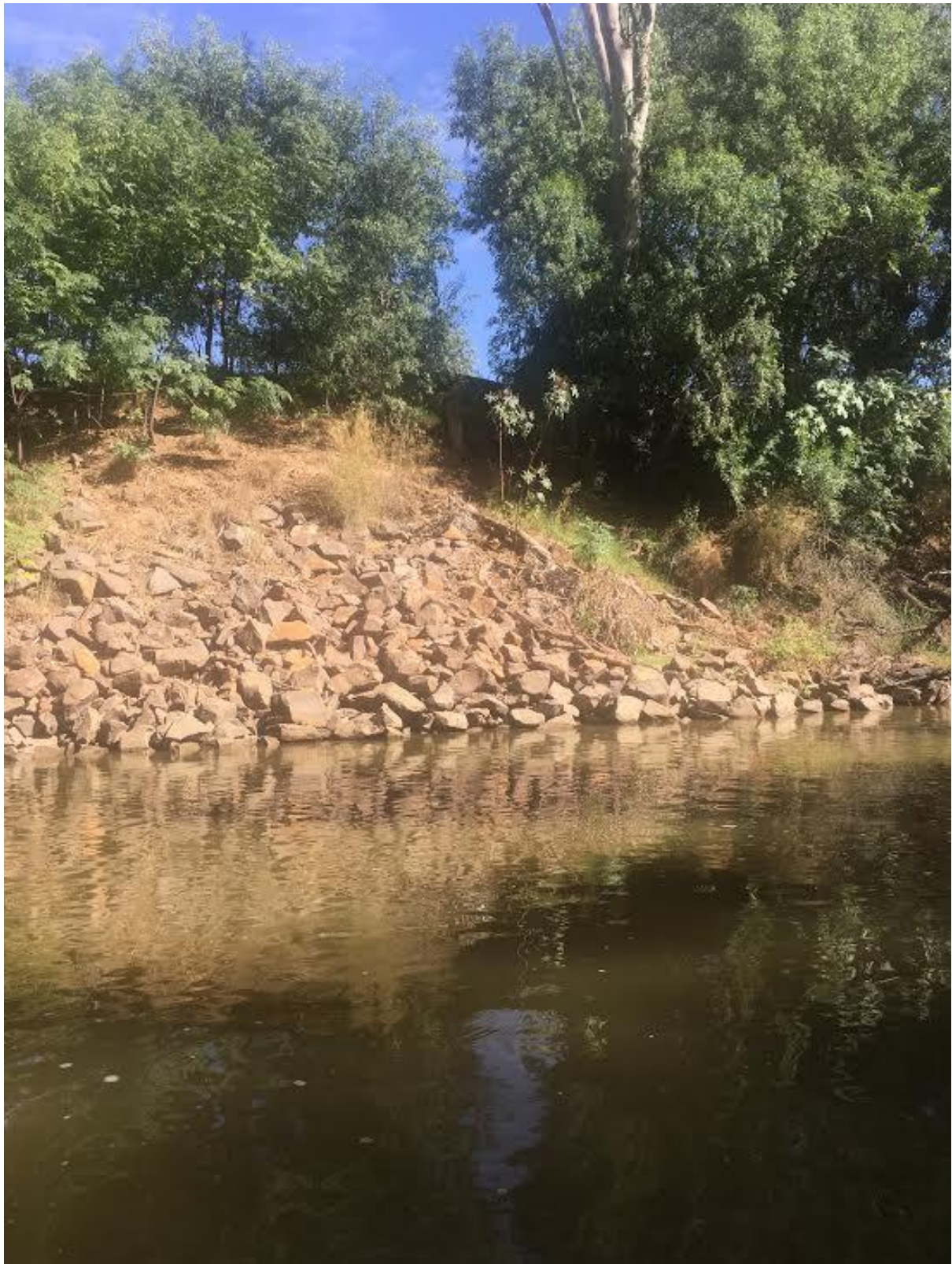
Photograph 25 Typical Rock Protection Elsewhere
