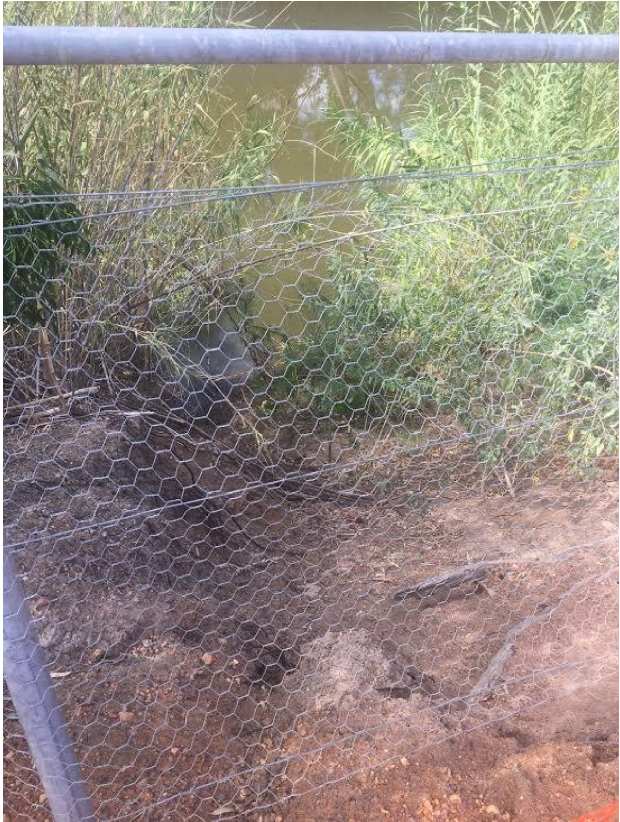
Photograph 8 Dentist Surgery/Courthouse Slippage
