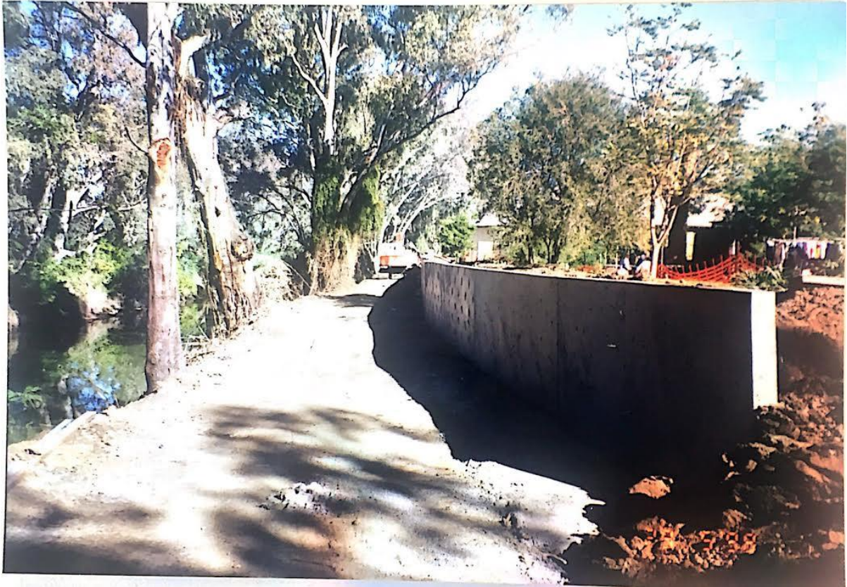
Photograph 22 Typical Retaining Wall Construction
