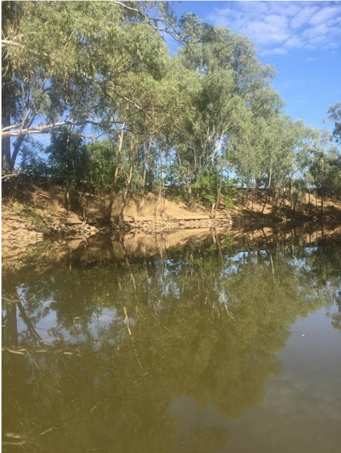
Photograph 14 Lions Park Sheet Pile Cap and Wall Riverside
