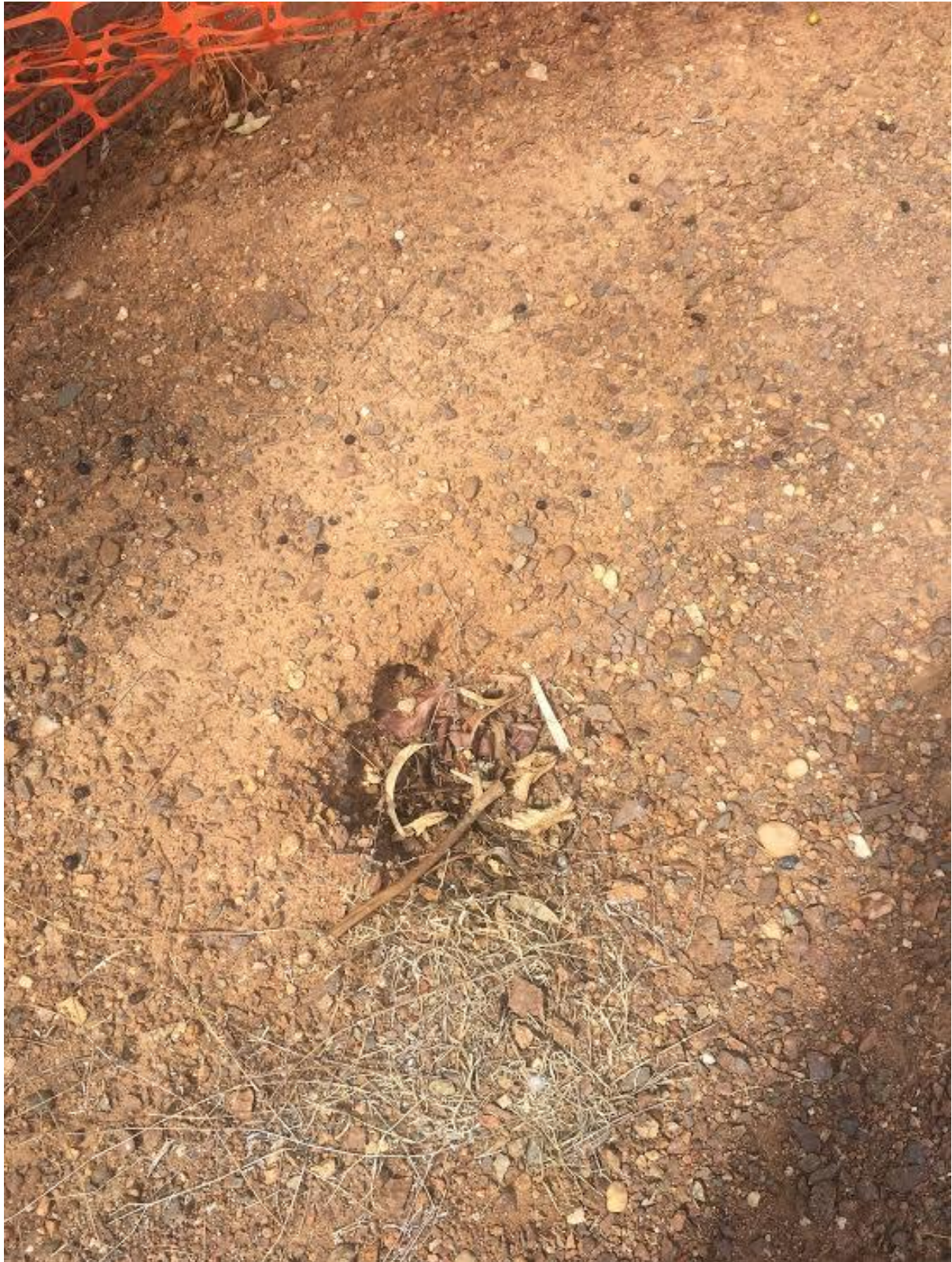
Photograph 11 Dentist Surgery/Courthouse piping
